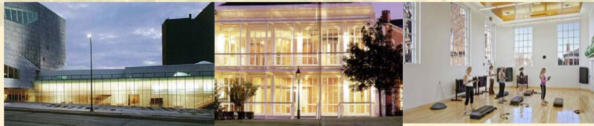
Recreation Addition with Transparent Facade
