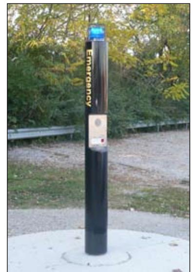
This is the first of a new model of emergency call box on campus. Standing 7 feet high, it is along Harrison Street west of Lynn Hall. High visibility is a priority, and Purdue will shift from this sample round pole to a square pole that more effectively displays "Emergency" facing all four directions.
