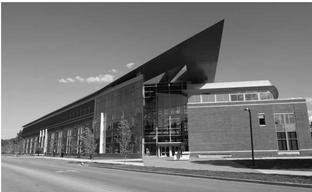
The Neil Armstrong Hall of Engineering
