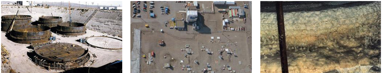
Hanford waste storage tanks during and after construction including one example of the waste stored inside a tank.
