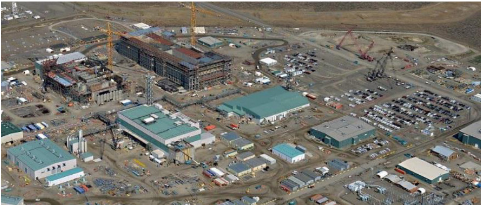
The Waste Treatment Plant (circa 2015) under construction at the Hanford Site.
