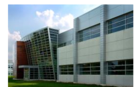
Birck Nanotechnology Center Clean Room Modernization and New Equipment
