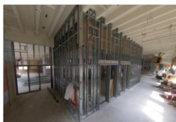
Mechanical Engineering Building Renovations
