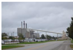
Chilled Water Capacity Enhancements
