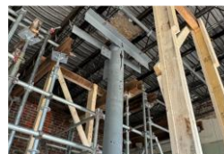
University Hall and Related Renovations
