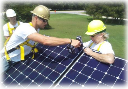
PV team installing panels during rebuild
