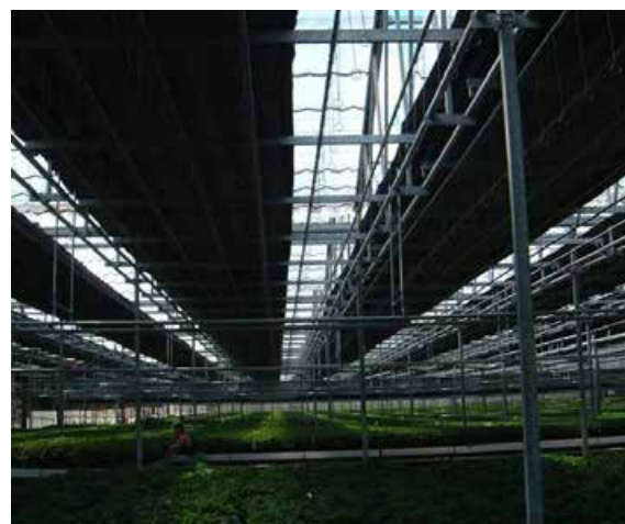
Figure 3. This blackout cloth curtain system encloses an entire greenhouse.
