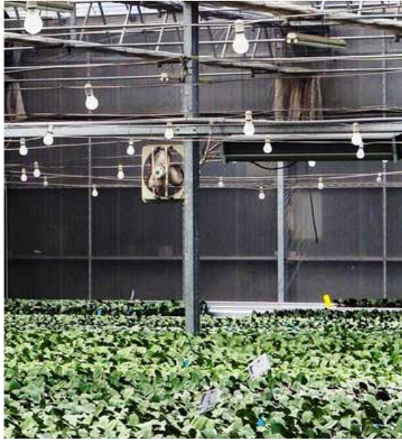
Figure 8. Incandescent bulbs are effective at providing long days, but they consume a lot of energy and are being phased out of production.
