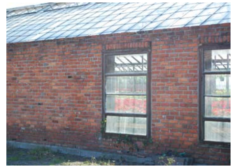
Figure 2. Heller's own brick and glass greenhouses.
