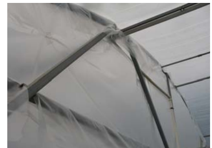
Figure 1. Sealing up gaps during the winter
