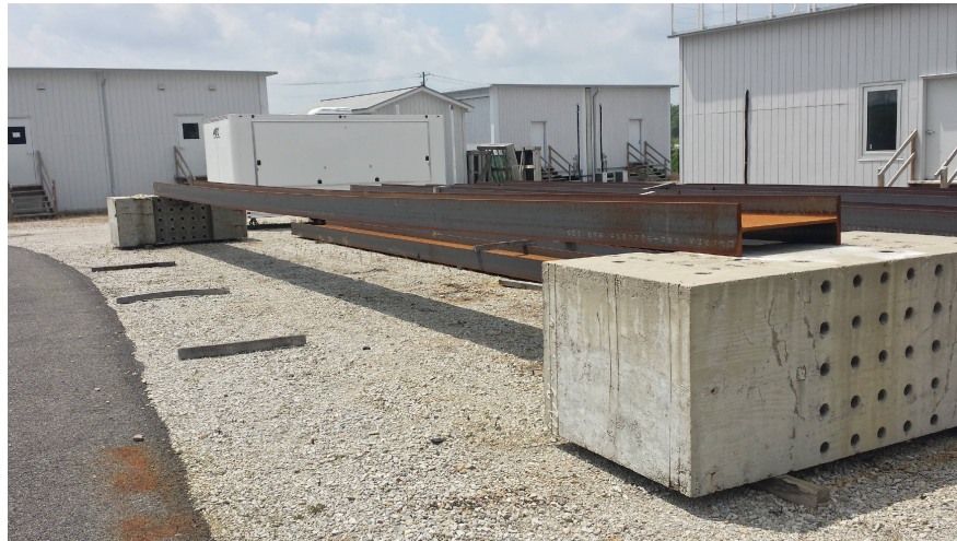
Fig. 6. Experimental setup of full-scale steel beam
