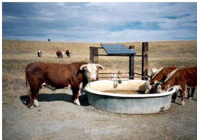
Figure 19. Solar-powered water pumping station. Source: NREL PIX.
