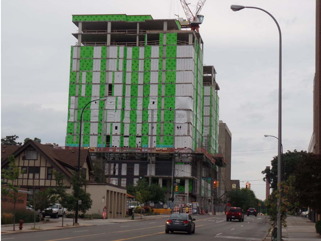
Figure 3: Site of 413 E. Huron Street (Photo credit: Louis Merlin 2015)
