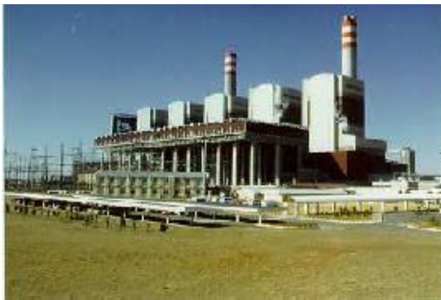
Figure 7. Majuba power plant ( http://www.eskom.co.za ).
