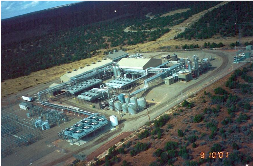
CO 2 Supply Operation McElmo Dome CO 2 Plant
