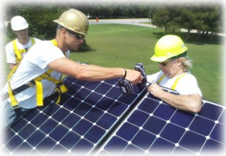
PV team installing panels during rebuild
