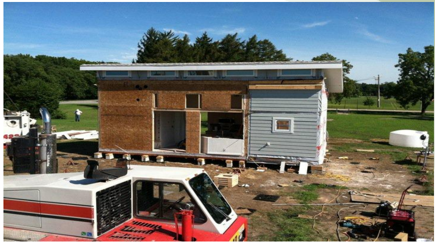
INhome mechanical core being craned off its base in West Lafayette
