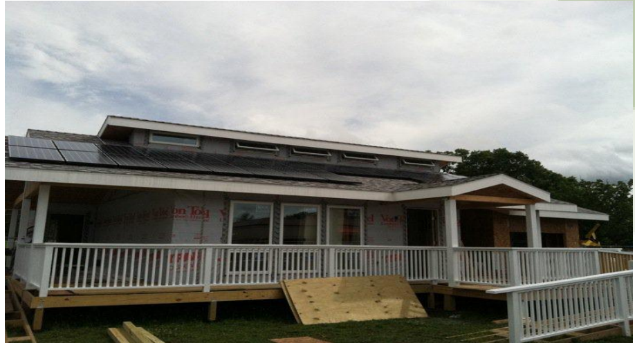
INhome under construction
