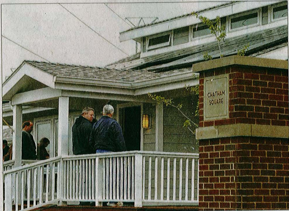
The Purdue INhome is on a permanent foundation — for the first time — at 1300 Shenandoah Drive in Lafayette. (PHOTOS BY BRENT DRINKUT/JOURNAL & COURIER)
