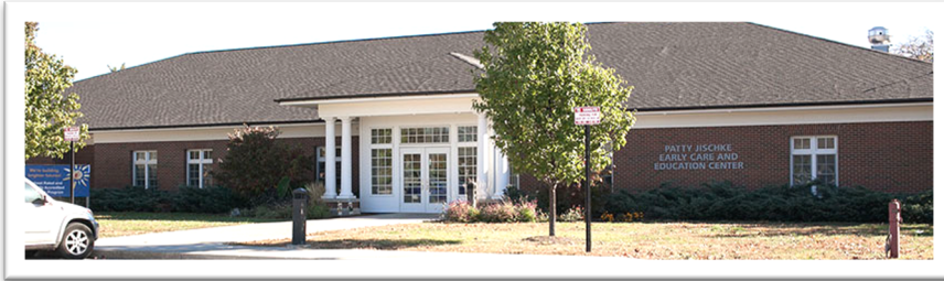
Patty Jischke Early Care and Education Center (Existing Facility)
