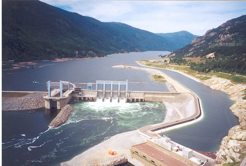
Figure 7-3: A run-of-river hydropower facility in British Columbia (Source: Clean Technica [8])
