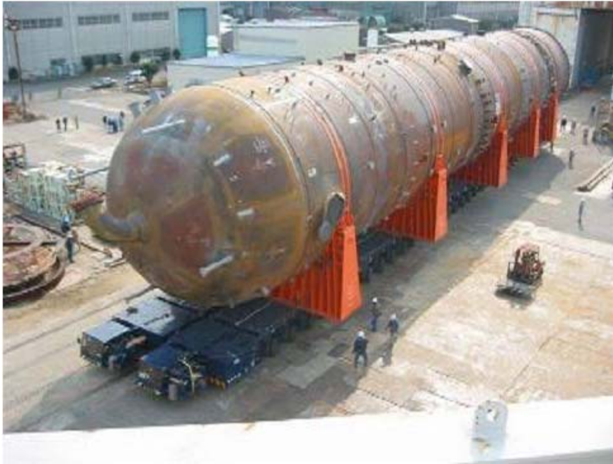
Figure IV.3. Onsite transportation of the Sasol FT Reactor for the Sasol Qatar Oryx GTL Plant (Louw, 2006. The capacity is 34,000 bpd, with 2 FT reactors; each weighs 2100 tons)
