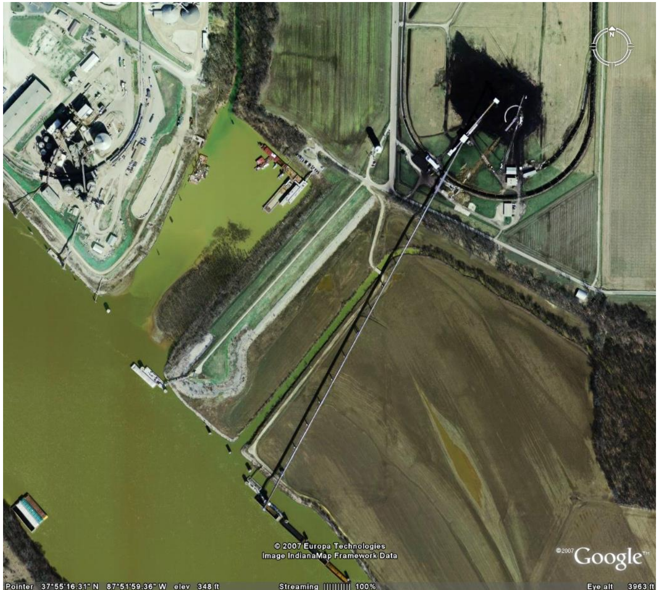
Figure XIII.7. Port of Indiana at Mt. Vernon Coal Handling Facility (Google Maps, 2007)
