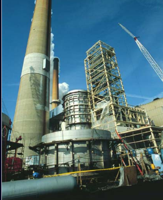
2001: Springfield's City Water, Light and Power Scrubber Installation ($17M grant)
