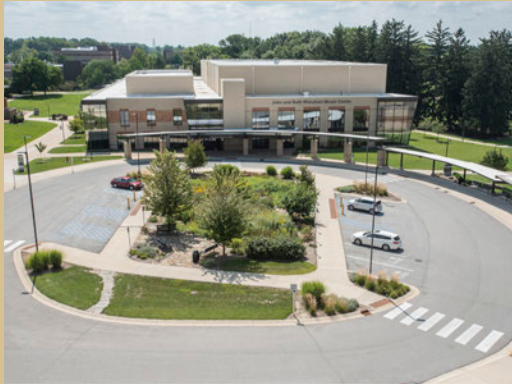
The Rhinehart Music Center drop-off was designed as a sculptural garden and a stormwater management system
