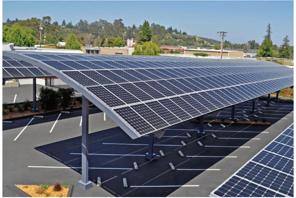
Land use can be optimized by installing photovoltaic shading structures on large surface lots to provide a source of renewable energy, mitigate the impact of heat island effect, and provide shade for humans and vehicles (Solar City JS Beam Carport Parking Structure)
