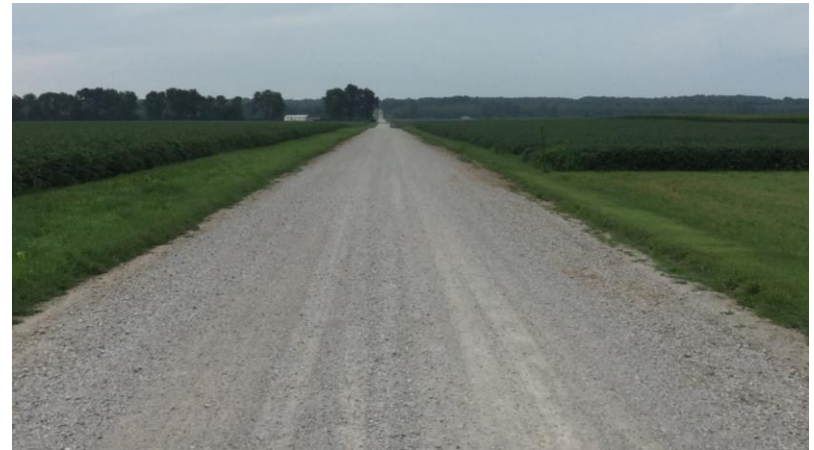
Both paved and unpaved roads need shoulder maintenance. Water cannot leave this unpaved road above so will likely cause eventual damage.
