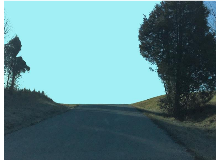
What's over this hill? Remind drivers to stay in their lane with a short centerline on each approach.
