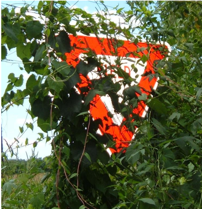
This Yield sign is completely covered so drivers do not know the other road has right of way.
