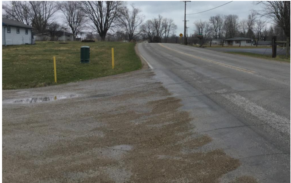
Sand on the roadway can interfere with vehicle braking and acceleration into traffic.
