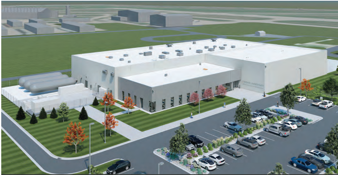
By 2023, the 65,000-square-foot, $41-million Hypersonics and Applied Research Facility is expected to be completed. It'll house the Hypersonic Pulse reflected shock/expansion tunnel (HYPULSE), donated by Northrop Grumman Corporation, and a newly developed and constructed Mach 8 quiet tunnel, which will be the first of its kind capable of collecting data at speeds greater than Mach 6.
